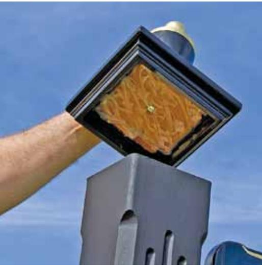
After spreading a coating of adhesive silicone on the inner cap's bare wood, we attach the fin/cap to the top of the detailed post, which is also bare to ensure a good bond.
