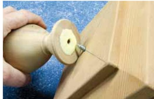
With yellow carpenter's glue at the finial base, to create a watertight fit, we tighten the lag from inside the cap.
