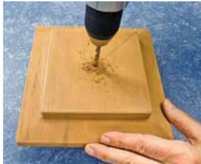
Using a 9/32-in. drill bit for a 1/4 x 3-in. lag screw, we drill a hole completely through the cap.
