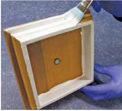
We apply three coats of primer to the finial/cap unit. We keep the inner base of the cap bare to allow better adhesion with silicone when it's installed on the post.
