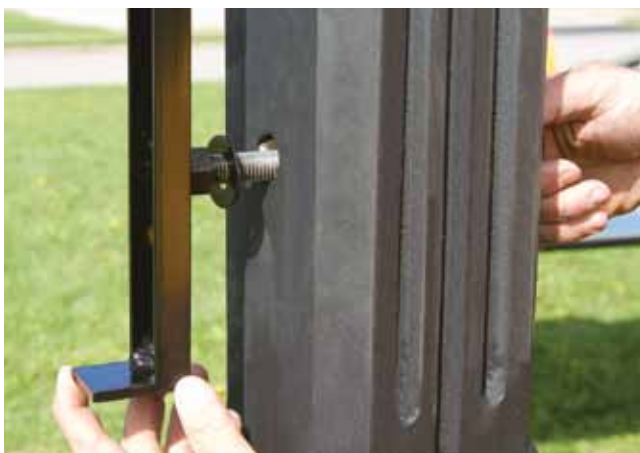
Because treated lumber can't be primed or painted, we stain our Southern-yellow-pine posts with a water-based stain. We apply two coats at the shop and a final, touch-up coat onsite after installation.
