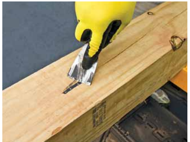
Using a putty knife, we spread the silicone deep into checks and around any knots, and let the silicone cure briefly.
