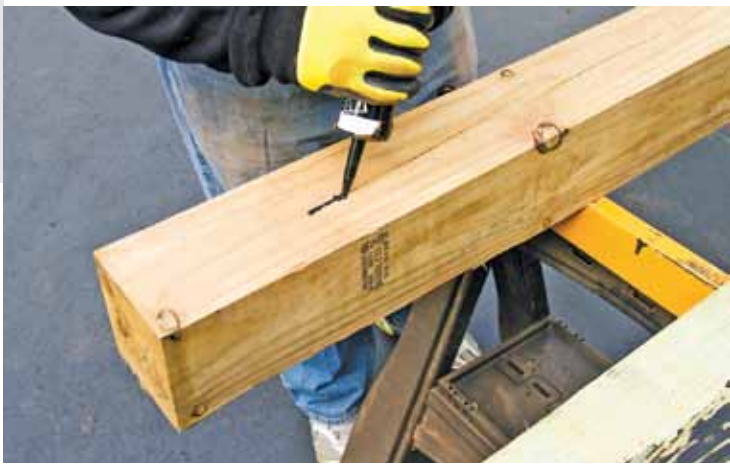
We select the best posts we find at the lumberyard, but they're often pretty unsightly. So, we seal cracks and splits by filling them with black-silicone caulk.
