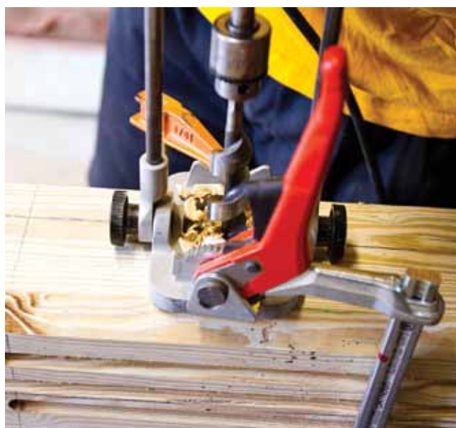
We clamp a perpendicular drill jig to the post and, with a 1-in.-diameter, auger-bit, drill completely through the post.
