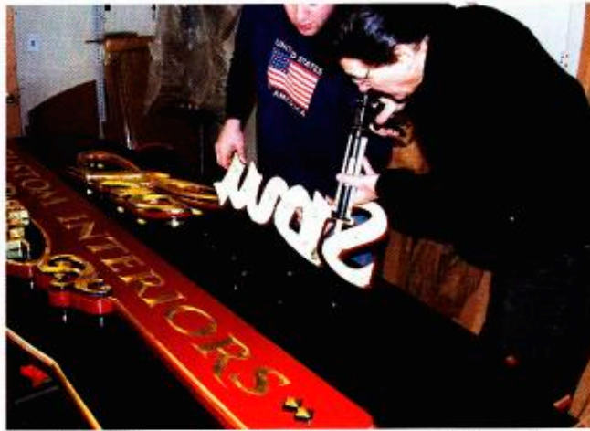
Francis and his son, Steven, applied the carved letters onto pre-drilled, silicone-filled holes within the Extira panel.
